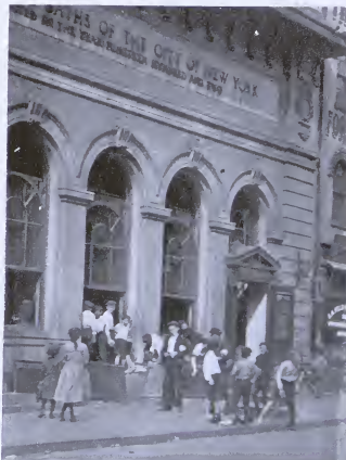
Public Bath, Ninth avenue and Forty-first street, located in conjunction with the A. I. C. P.
